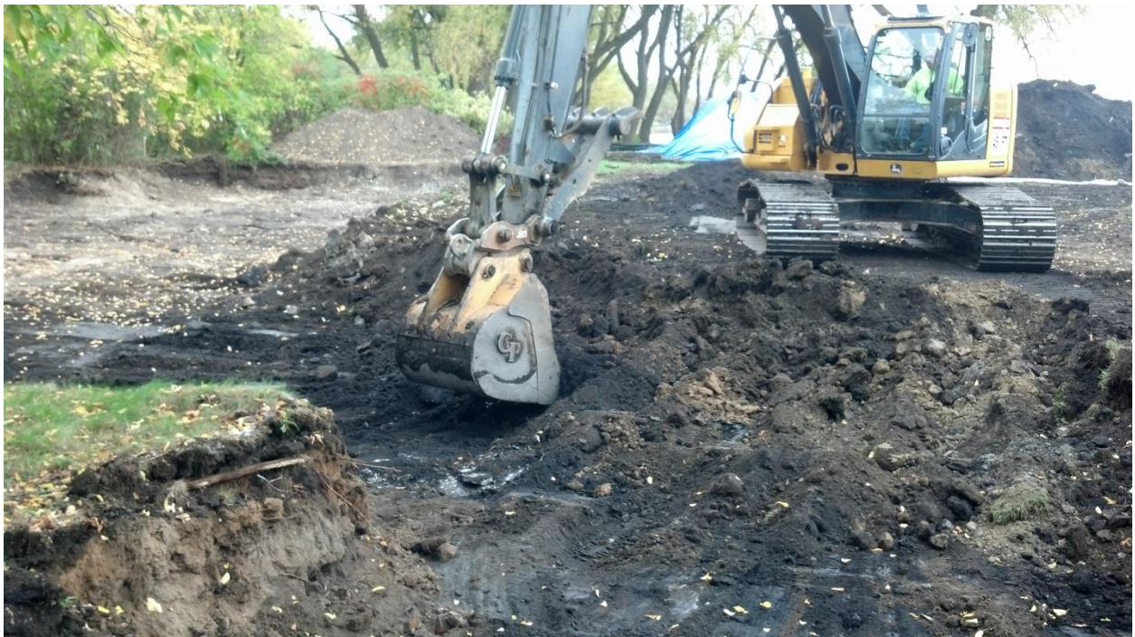
Photo 3: Excavation of contaminated fill soils by backhoe in the central portion of the monitoring area.
