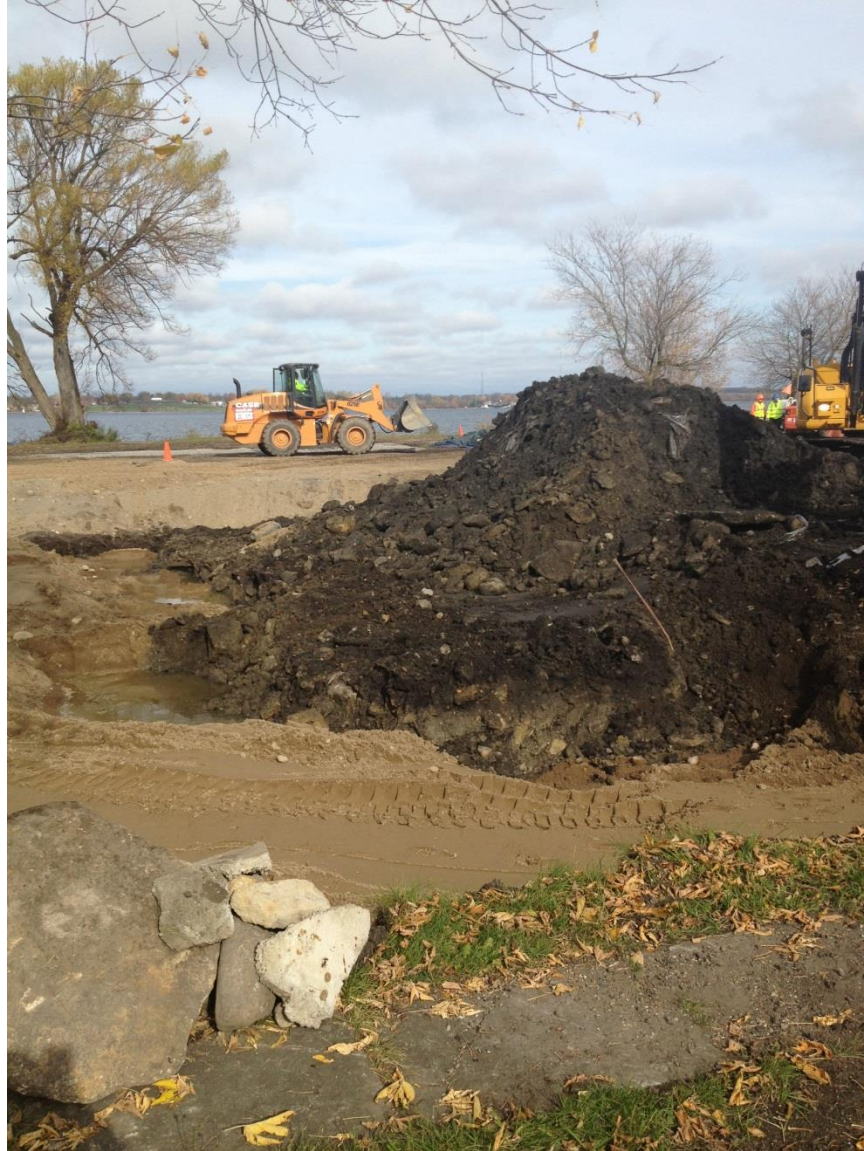
Photo 27: Central section of the archaeological monitoring area facing north. Note the subsoil present at the base of the unexcavated section indicating total excavation depth exceeding 1.5 m (5 ft).
