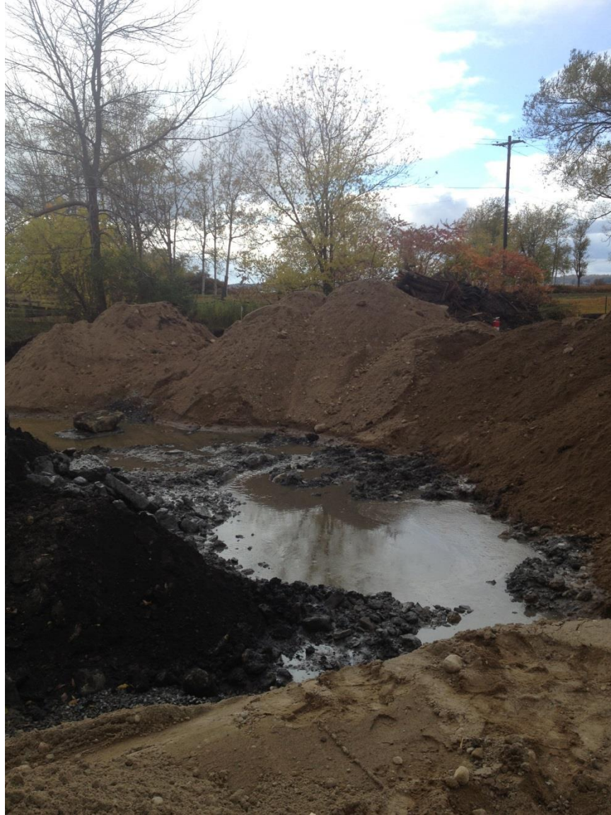
Photo 6: Clean fill deposited in excavation area after removal of contaminated soils. This is in the eastern section of the monitoring area.
