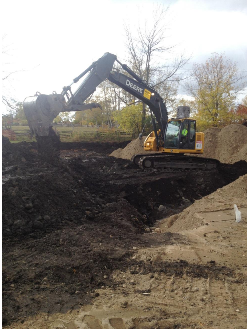
Photo 16: Mechanical remediation in the northwestern section of the archaeological survey area facing northwest. The final depth of excavation is depicted here. Its depth is suggested by the position of the backhoe, sitting atop the initial excavation surface 0.9 m (3 ft) below the ground surface, and its relation to the clean fill.
