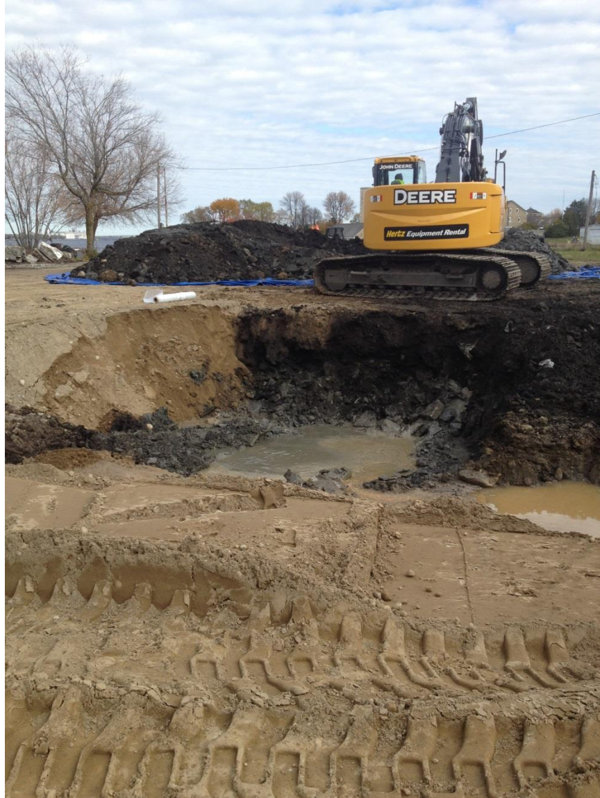
Photo 32: Eastern edge of excavation in the archaeological monitoring area showing one of the deeper areas, approximately 1.5 m (5 ft) of excavation.
