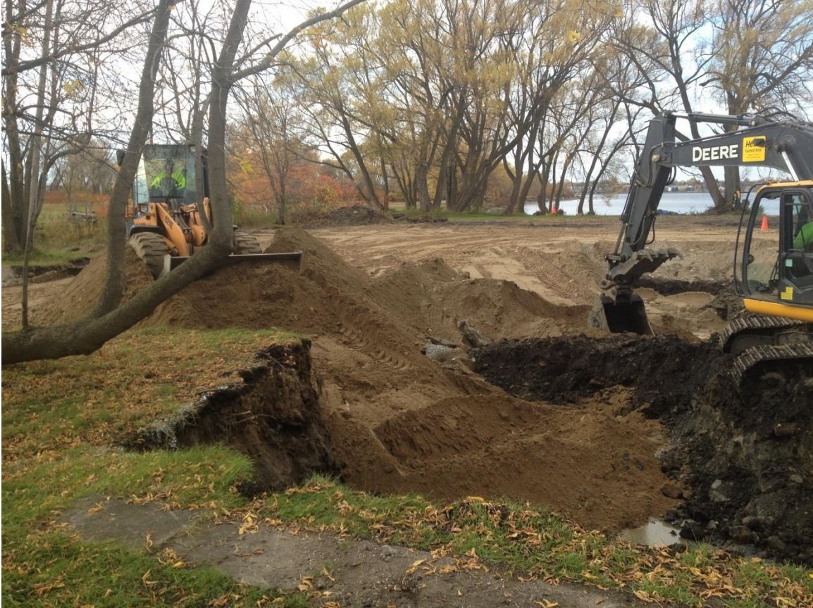
Photo 7: Placement of clean fill in excavated area along the southern edge of the monitoring area.
