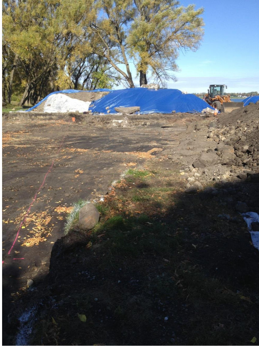
Photo 4: East-central portion of the monitoring area partially excavated. Note covered piles of excavated soil awaiting removal from site.
