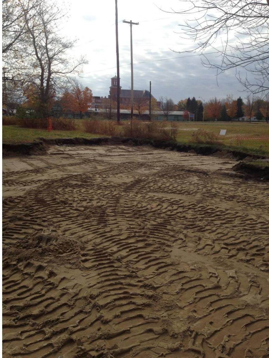
Photo 9: Southwestern corner of the monitoring area nearly backfilled with clean soils.
