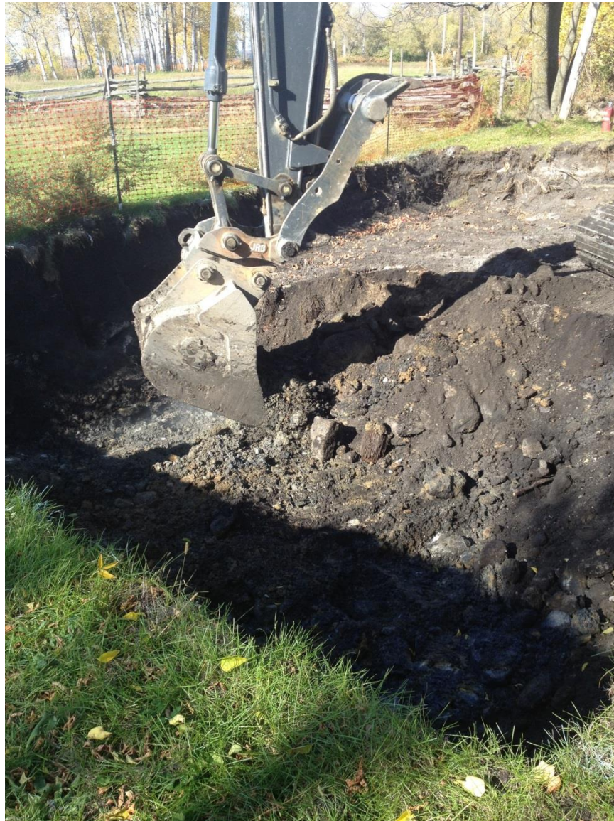
Photo 12: Continued excavation below the 0.9 m (3 ft) initial excavation in the southwestern corner of the archaeological monitoring area.
