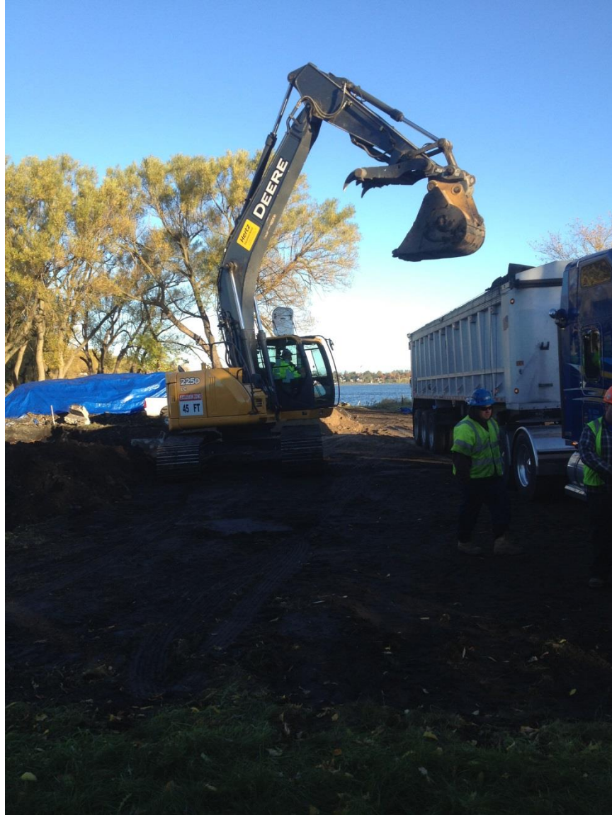
Photo 5: Loading contaminated soils into truck for removal from site.
