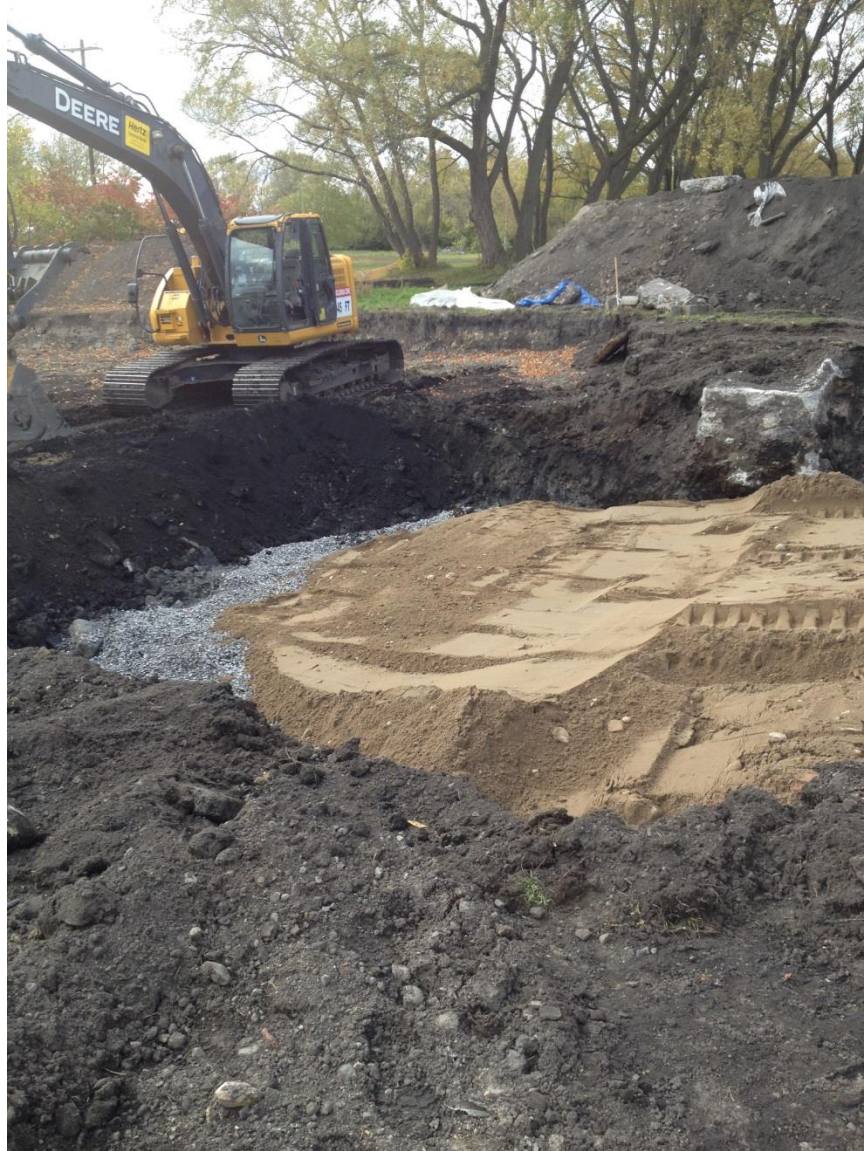
Photo 8: Clean fill atop crushed stone layer in the north-central portion of the archaeological monitoring area. Crushed stone was added as base in particularly wet areas. Note the concrete feature on right side of photo.
