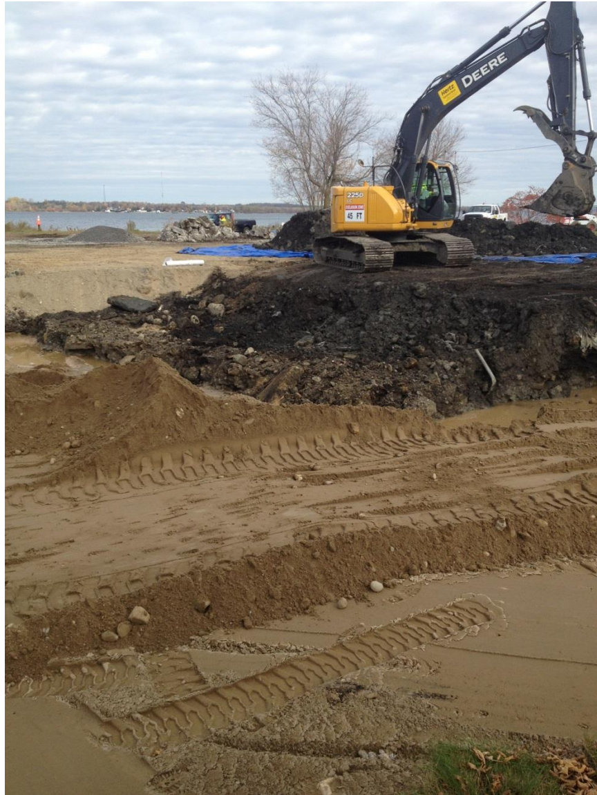
Photo 34: Eastern end of the archaeological monitoring area nearly filled with clean material, facing northeast. Note the depth of final excavation depicted by the east wall profile and grey-brown subsoil at its base.
