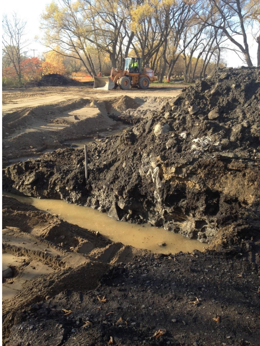
Photo 19: Deeper excavation in the southern end of the archaeological monitoring area facing northwest. Note the depth of the clean fill relative to the grey-brown subsoil visible at the base of the unexcavated soil in the center of the photo.
